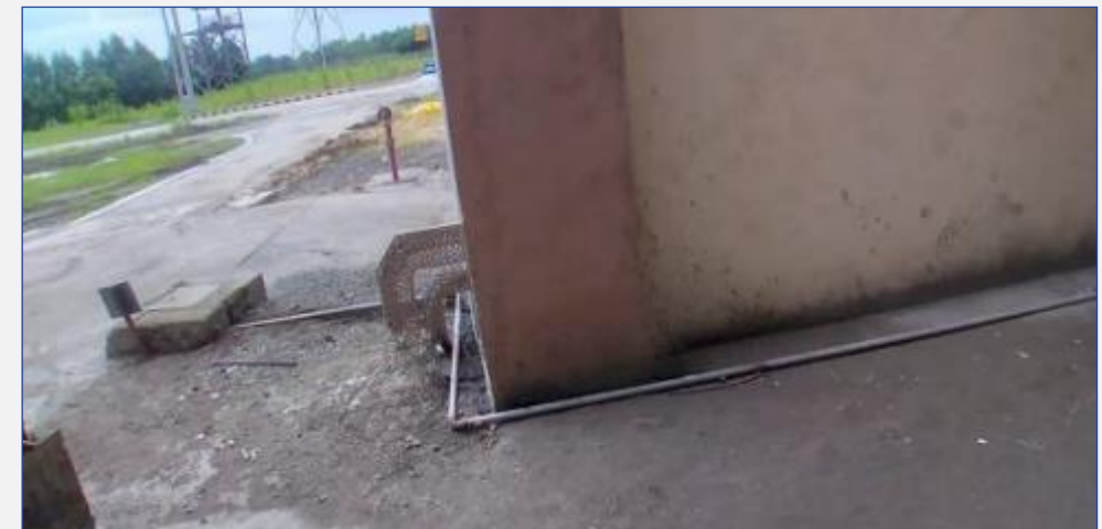
◆ Pipe lines connected to Earth pits ◆
