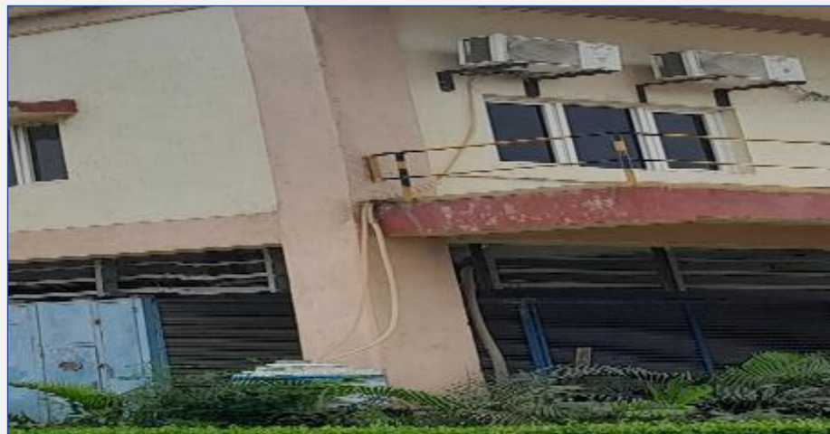
◆ Drain Water collection from AC ◆
